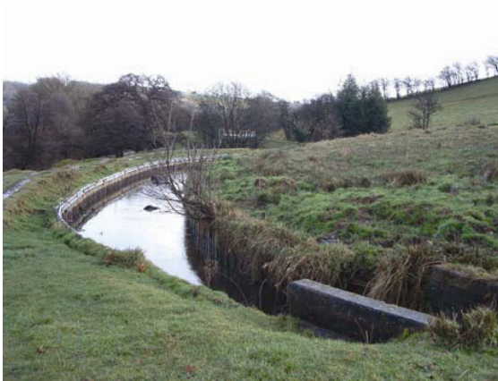
Canal feeder and culvert
