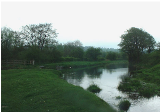
View from feeder to Barnfields Aqueduct.
