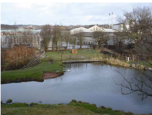
Existing terminus of Leek Arm at aqueduct.
