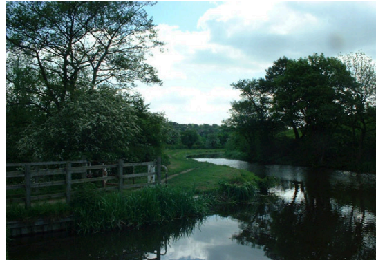
View east along canal from aqueduct.
