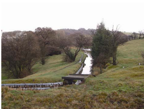
View east along canal feeder towards aqueduct
